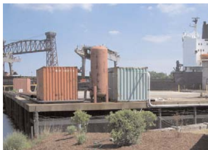
A stormwater management system was developed for all barges including inspections.
