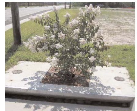
Tree box filters not only improve stormwater runoff, but the rain helps water the tree!
