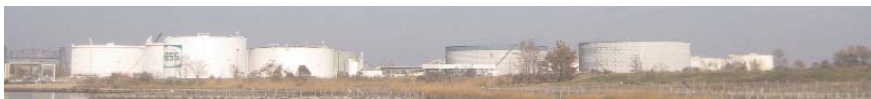
Hess, a key partner in cleanup efforts at Money Point, reduced air emissions by 5,468 tons.
