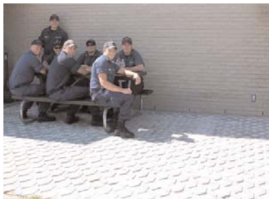
Permeable pavers help prevent stormwater runoff from reaching the river.
