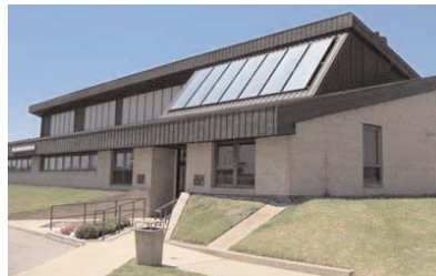
ISC in Portsmouth has installed seven solar panels on the community services building.
