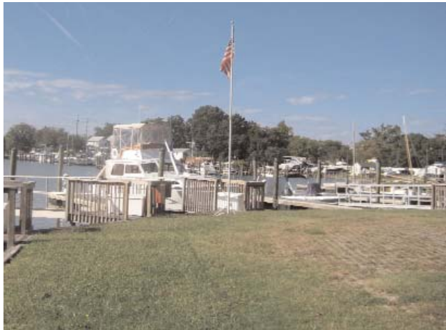
Knitting Mill Creek Yacht Club's driveway, parking lot and walkway are all green! The permeable pavers used allow grass to grow in between and not only look green (above), but also absorb rainwater.
